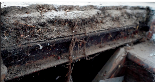
Figure 15. Metal elements of the jack arch flooring and cement plaster
