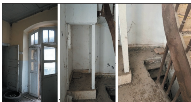
Figure 11. Z01 the passenger reception and Z04, the traces of wet volume added and the staircase
