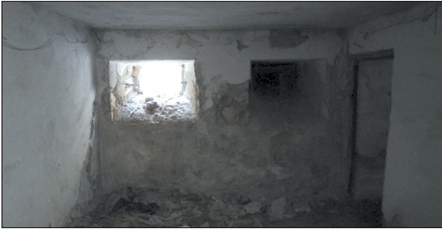
Figure 13. Basement floor areaway windows
