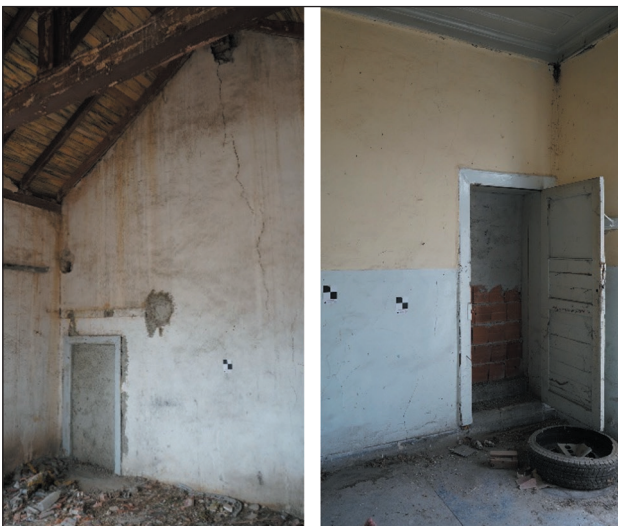
Figure 21. The door connecting Z05 with space Z06 was closed by building a wall.
