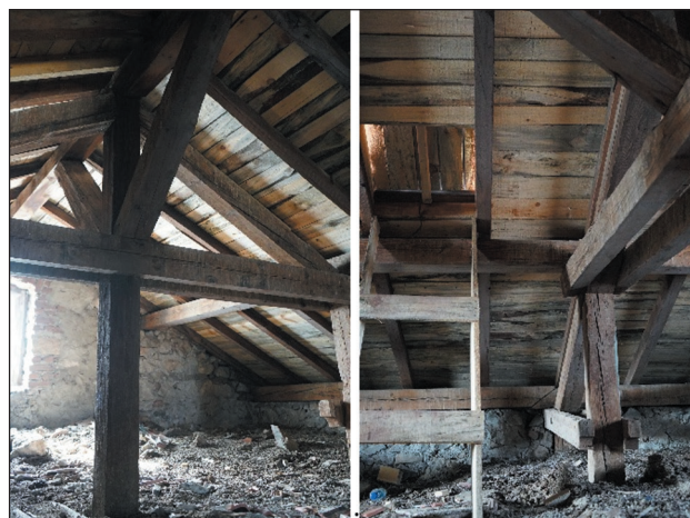
Figure 9. Building roof after simple repair
