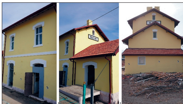
Figure 7. Facing the platform and short side façade
