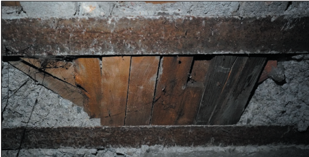
Figure 14. Metal elements of the jack arch flooring
