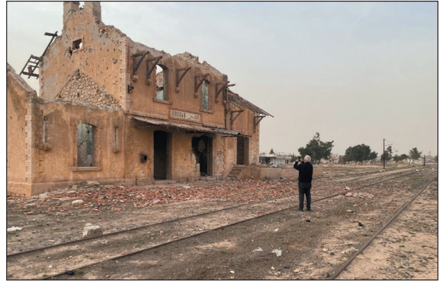
Figure 2. Halep, Koussair station (2024)
