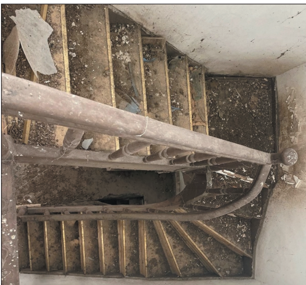
Figure 16. The staircase and upper landing
