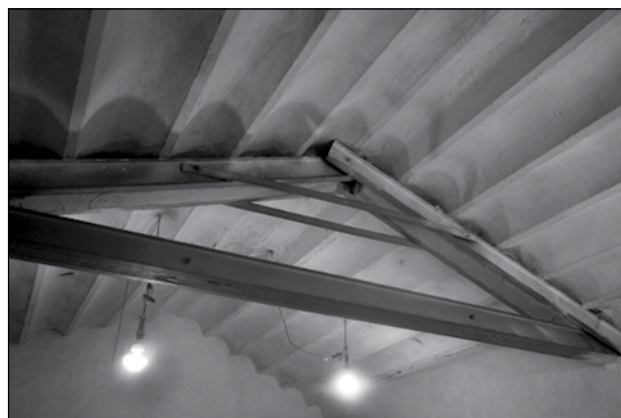
Figure 2. In a building built after the 1908 fire using jack arch for roof construction
