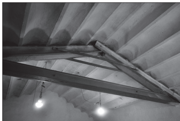
Figure 2. In a building built after the 1908 fire using jack arch for roof construction
