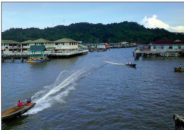
Photo 5. As part of the pilot rejuvenation project in Kampong Lurong Sikuna uniform style similar to land-based housing estates https://commons.wikimedia.org/wiki/File:Kampong_Ayer_BSB1.JPG
