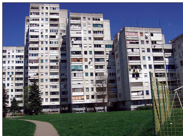
Figure 5. Residential settlement “Borik” - Banja Luka. [4]
