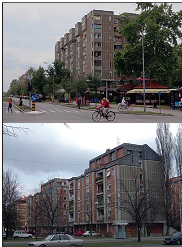
Figure 12. Residential settlement “Limak 3” in Novi Sad, photos of realized buildings. [4]
