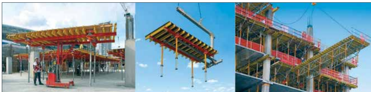
Figure 6. Table Formwork [8]
