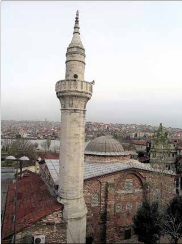
Figure 6. The dome, outer portico, and minaret of the Atik Mustafa Pasa Camii are the Ottoman period additions to the structure (Esmer, 15.12.2009).
