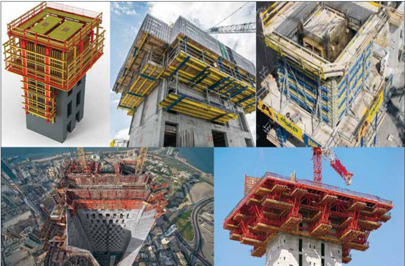
Figure 5. Self-climbing Formwork Platforms [8]
