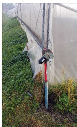
Figure 8. Position of the ventilation mechanism on the greenhouse
